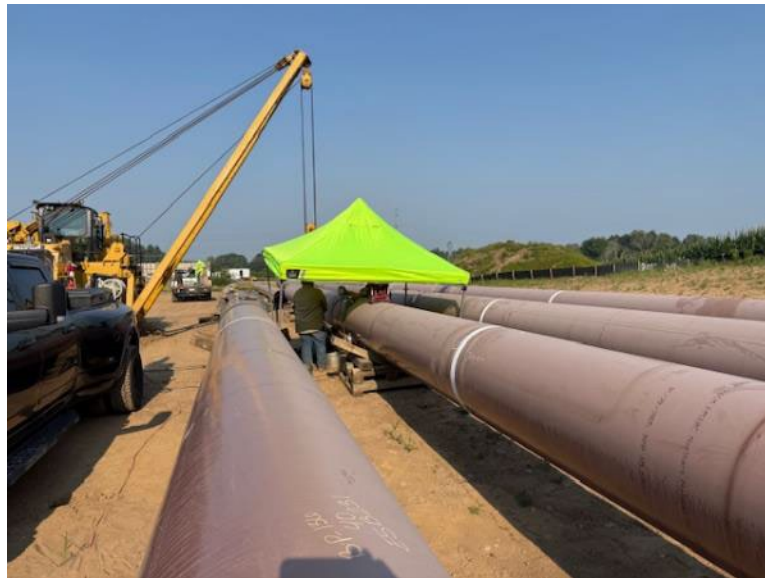
Facing west near MP 1.35, welding bore pipe ongoing
