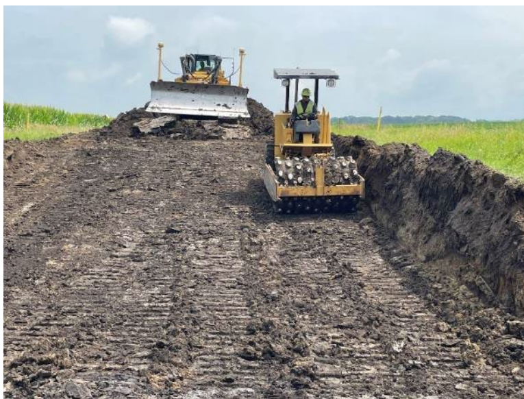
Facing west at MP 33.19; Jensen backfilling and compacting the County Road 80/154th Street crossing
