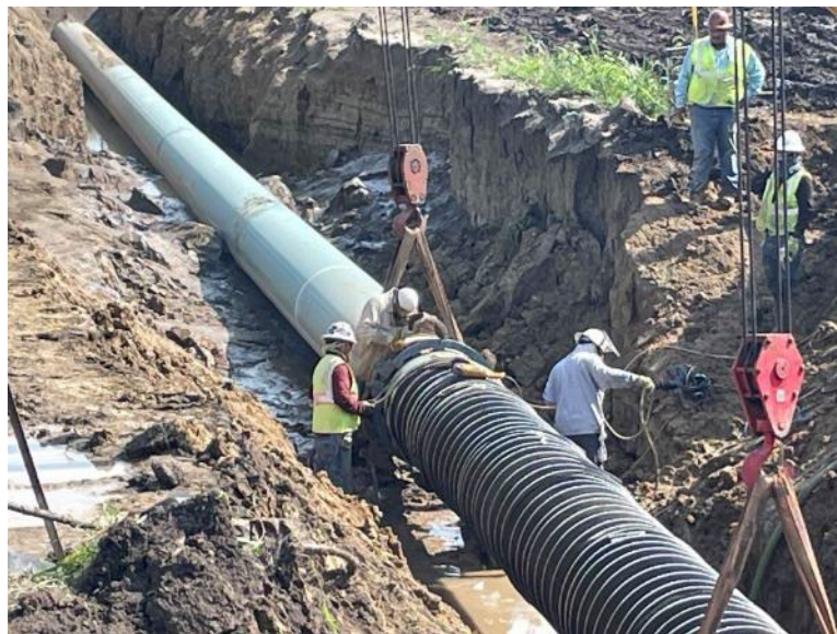
Facing southwest at MP 33.18, K&K lowering-in and tie-in at the County Road 80/154th Street crossing
