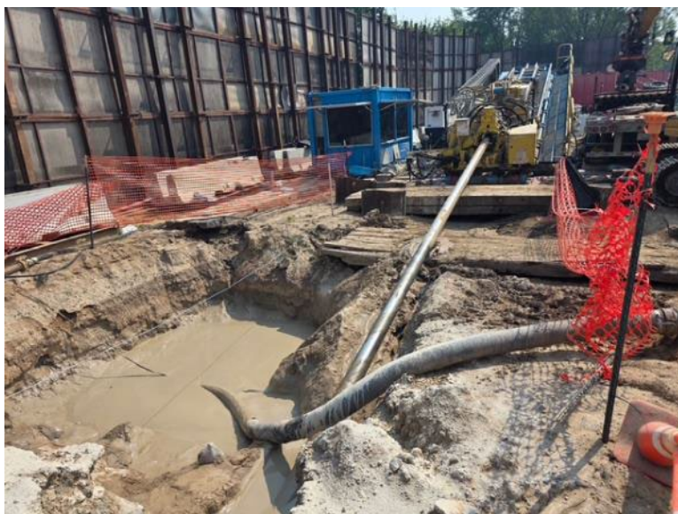
HDD P4-5, continued the pilot pass
