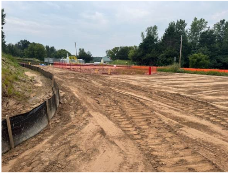
Facing south near MP 1.0, removal of short segment of existing pipe to accommodate HDD activities and backfill completed
