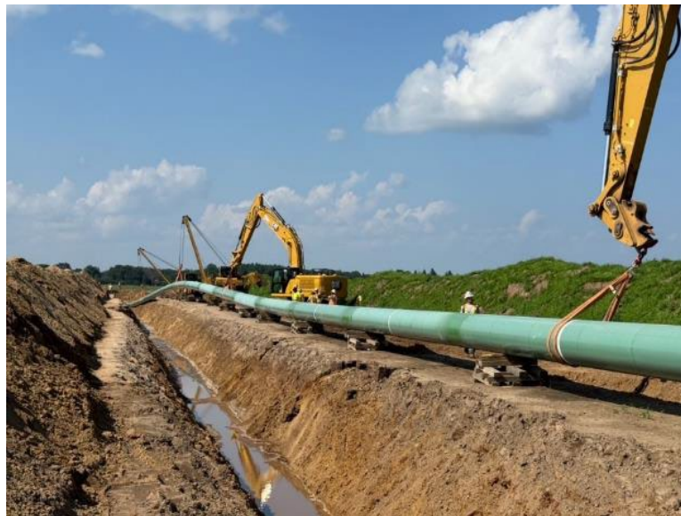
Facing north, Otis lowering-in the line pipe near MP 1.6
