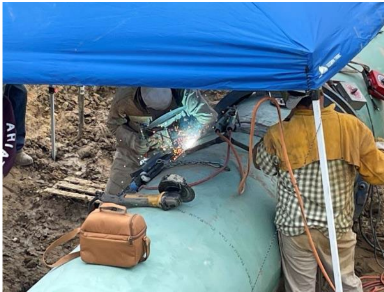
Facing northwest at MP 32.65, K&K welding mainline pipe north of 140th Street
