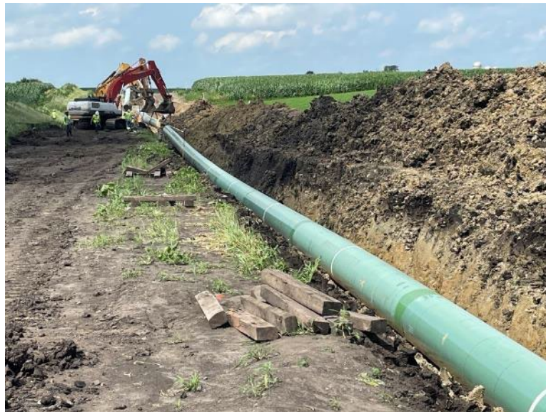
Facing north at MP 32.0, K&K lowering in mainline pipe north of County Road 80/154th Street
