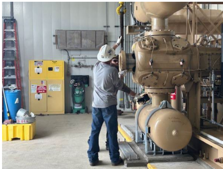
Facing west, Archrock removing compressor head
