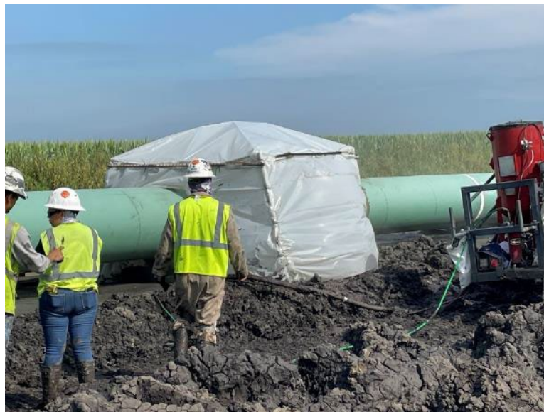
Facing northwest at MP 33.55, K&K sandblasting and coating mainline pipe south of 165th Street
