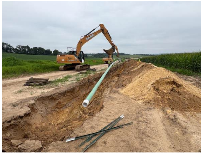
Facing east near MP 3.3, contractor lowering-in pipe
