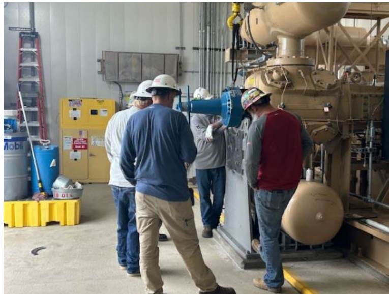
Facing west, Archrock installing new compressor head
