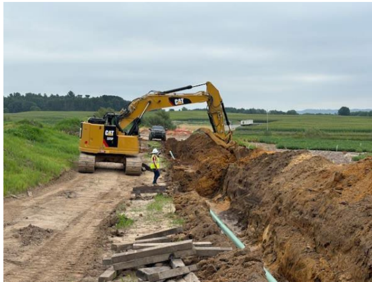
Facing east near MP 3.4, contractor backfilling ditch line
