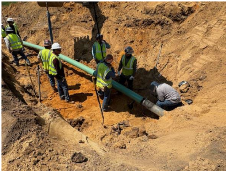
Facing southeast near MP 2.55, contractor completing tie-in
